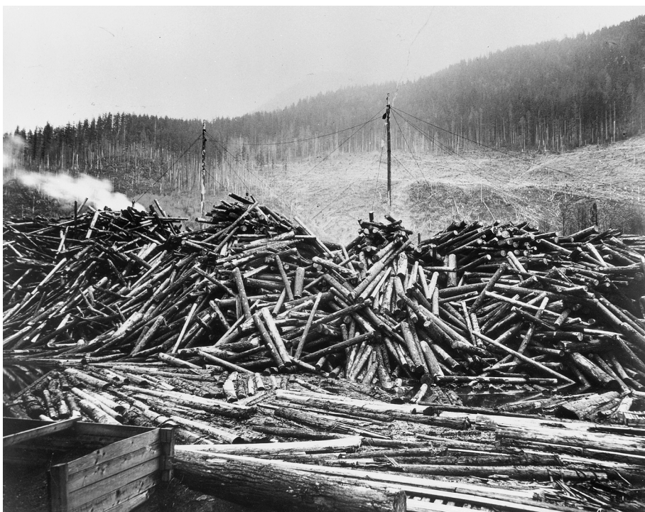
Yarding logs with spar trees, Bloedel Donovan Lumber Co., Skykomish, Washington, date unknown. Negative no.: UW 1695. Photo: Darius Kinsey. Courtesy University of Washington Libraries
